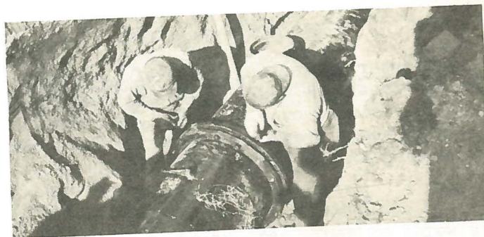
Bolting up one of the 24" C-N joints.
