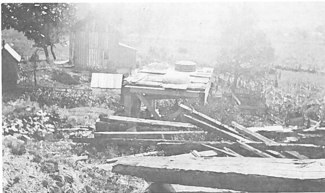
The house and the ruins of the old mill, once owned by Nathan Wright, Sr. Located in Bedford County, Pennsylvania, near Centerville; halfway between Cumberland, Maryland, and Bedford, Pennsylvania
