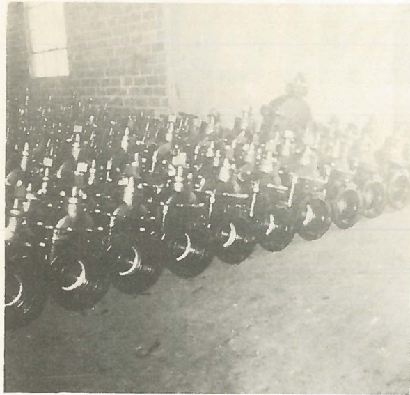
Two views of our Iowa valves, with the new "O"-ring packing, ready for shipment. There has been a great amount of work necessary to develop this design and we think it adds to the appearance of the valve.
