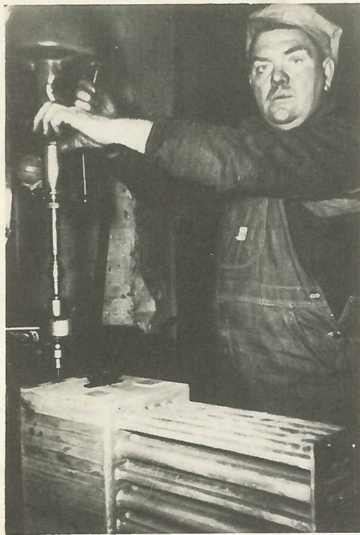
John Hall, Unit Heater Assembly, drilling a unit heater casting.
