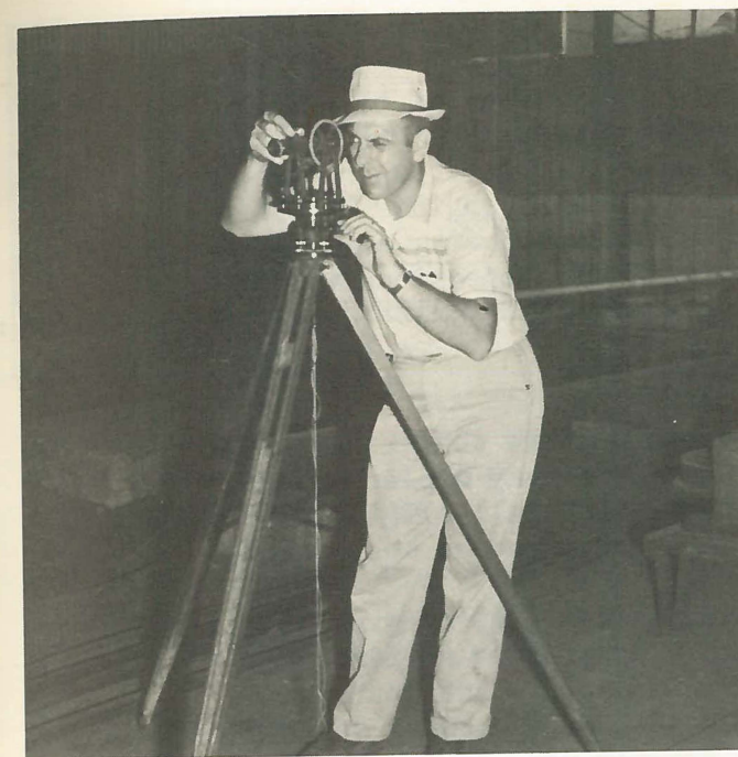
Gene Love, Engineer, is shown lining up anchor pins for the foundation for #5 machine through a transit.
