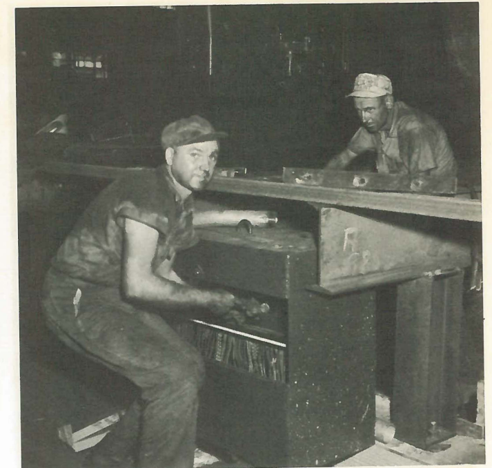
Toby Blair and John Hubbard, Electricians, are shown rewiring a junction box to #4 machine. "Man, how do you know which wire goes where?"
