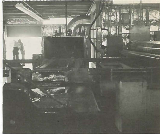
Above is a view of the seal coat machine recently installed at Bensenville.
