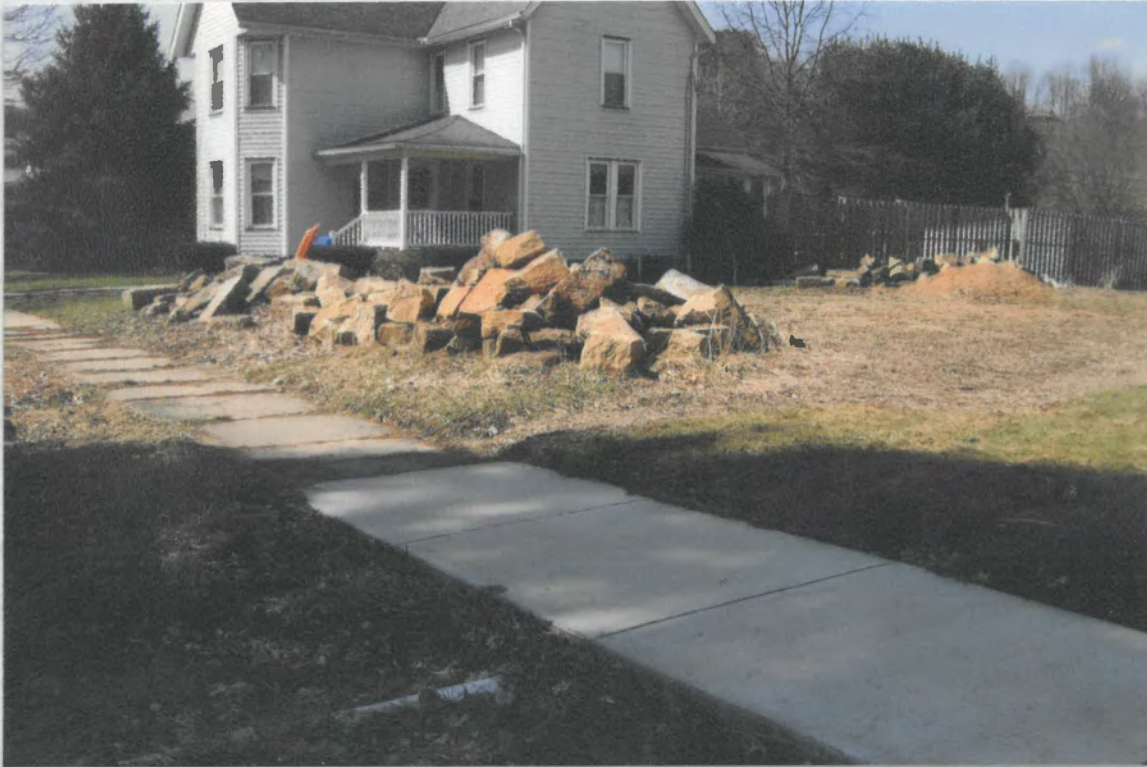
Foundation of former Rippeth Family home - photo taken 1-2008 Looking north-west.
