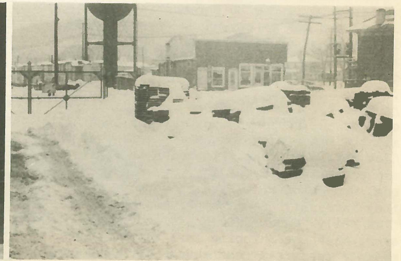
There are flasks and bottom boards beneath the snow.
