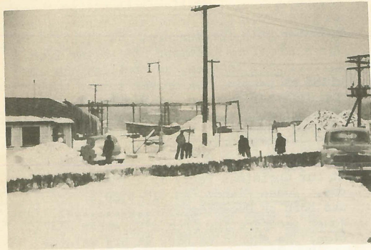
Monday, November 27th - Digging out the main gate on State Street.
