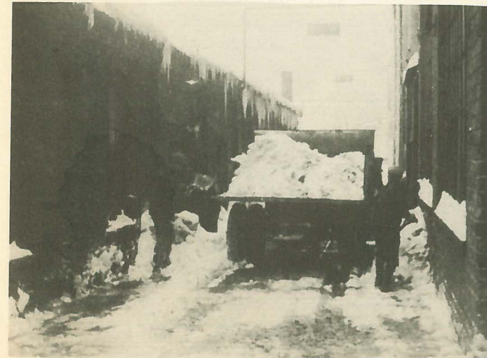
Our Chevy truck and a gang of fellows clear the roadway between the Power House and the Machine Shop.
