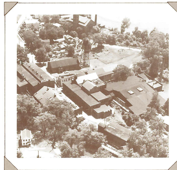
Aerial view of the Eddy Valve Company, Waterford, (Albany) New York
