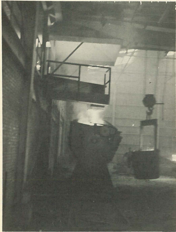
RECENT HOOD INSTALLATION
