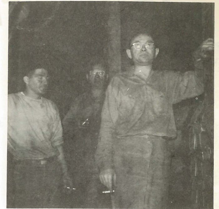
JOE FRANCESCONI, LOUIE JANKOWSKI, and JOHN BAYLAK take a break from their work on the wheelabrator.
