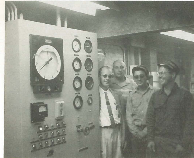
POWER START UP FOR CUPOLA HOT BLAST
