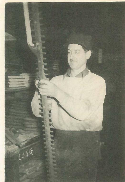
Harold "Hats" Meeks, Cores, files one of the long 19-section Burner cores. It takes good eyes and steady hands to file one of these sections without breaking those fingers off.
