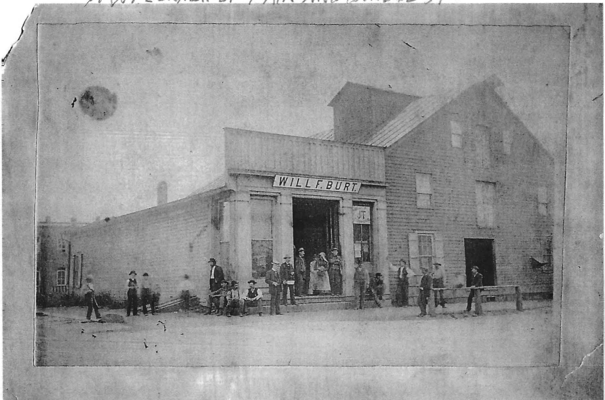
S. W. CORNER OF MAIN AND BRIDGE ST
