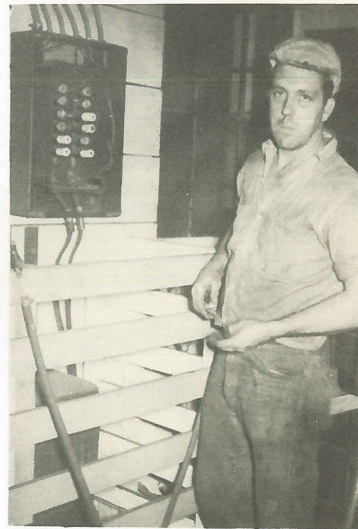
Richard McMillen doing a little electrical repair work in the Unit Heater Department.
