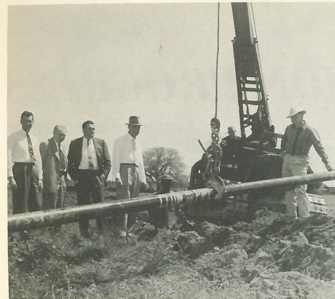
Laying the first Clow Bell-Tite pipe at Houma, Louisiana in May 1957.
