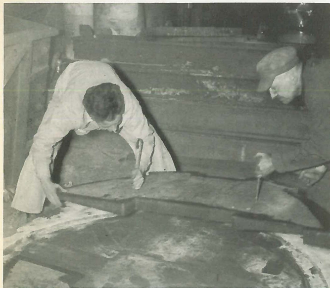
LEO PATNODE and HARRY HABURA lift a section of pattern from a gate mold.
