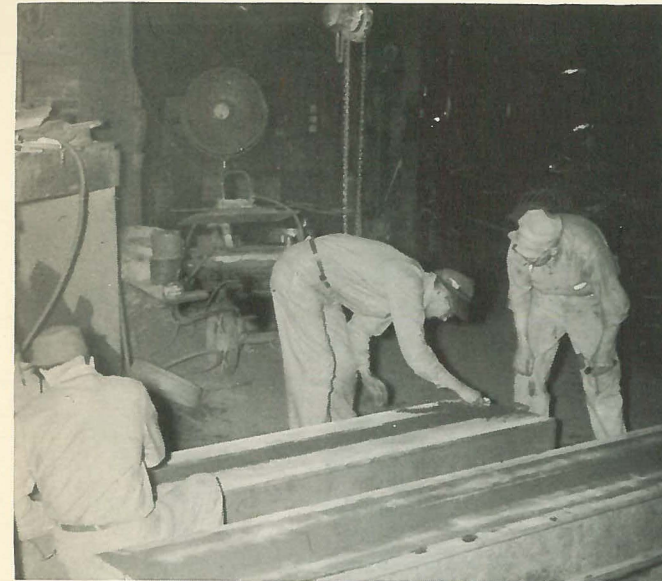
The last minute preparations are made readying one of the molds for the bronze stem.
