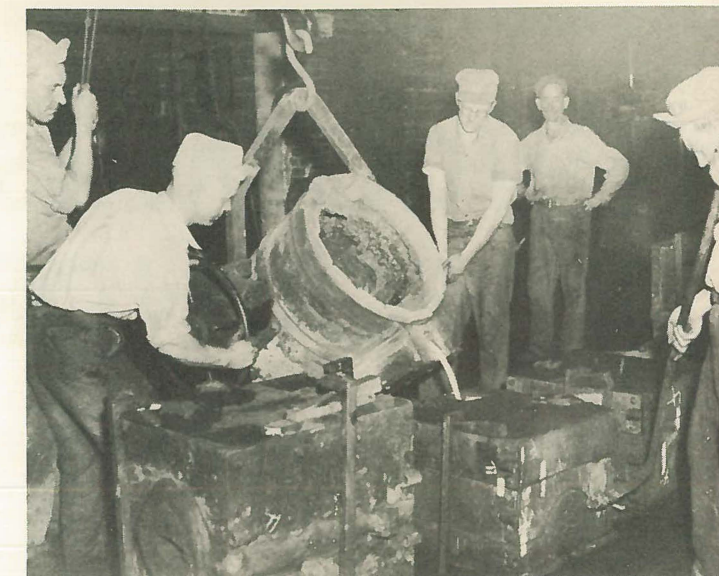
Pouring a number of castings at Iowa Valve.
