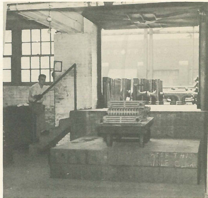
HYDRAULIC PLATFORM LIFT permits push-button control to move loaded platform truck to storage yard level.
