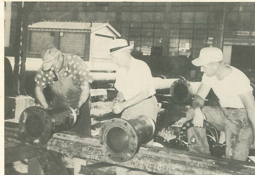
Talmadge Foote, George Little, and Howard Bryant are inspecting flange pipe.
