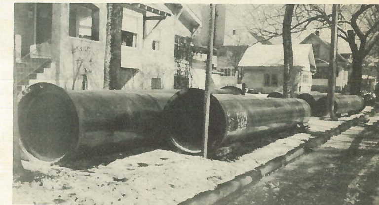
Above, Clow cast iron pipe ready for installation. Below, a length about to go into the trench that has been dug.
