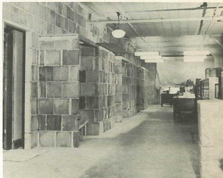
Tile blocks, used to partition off the executive office rooms, have now been plastered and painted. The protruding area will be used for file cabinets and closet space.
