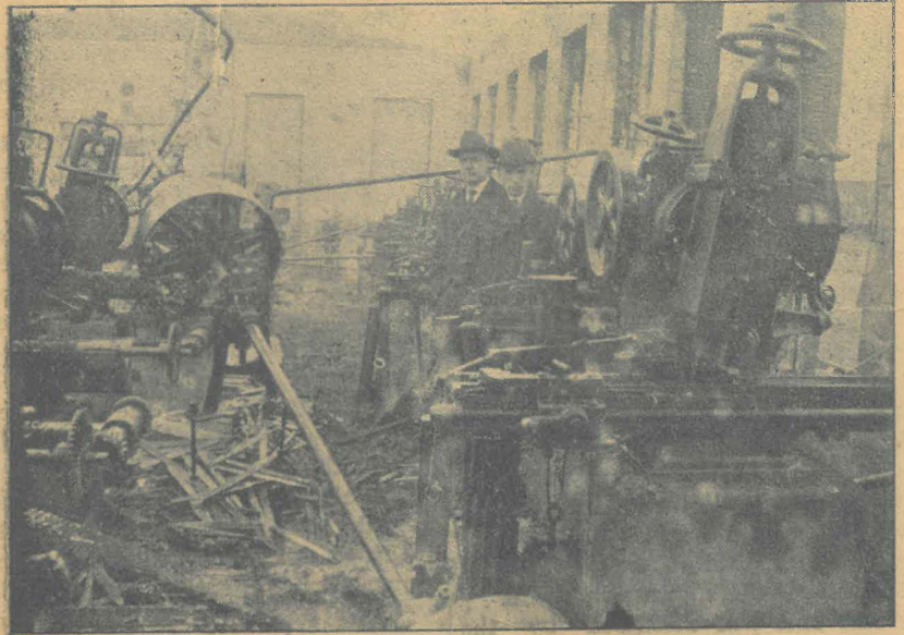
Remnants of the Rex fire, showing the boiler and other machinery, as they were salvaged from the ruins of the building.
