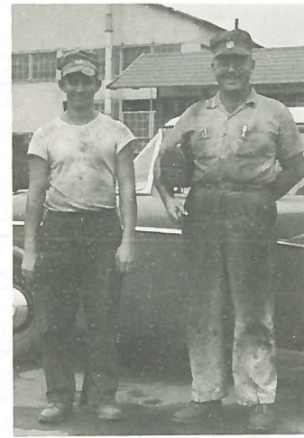
DWIGHT SELF, Carpen- ter Pool; EWIN SELF Electrician.
