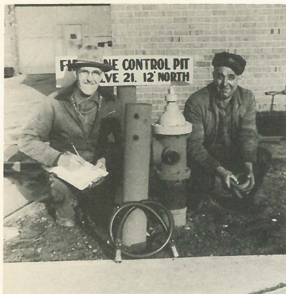
Cliff Williard of the Pattern Shop and Art Conard of Maintenance are completing a fire and sprinkler inspection.
