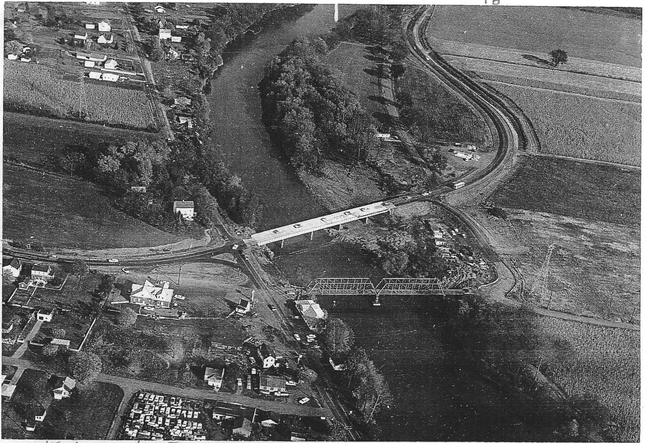
NEW CONCRETE BRIDGE BUILT IN 1961 PILLING ST.
