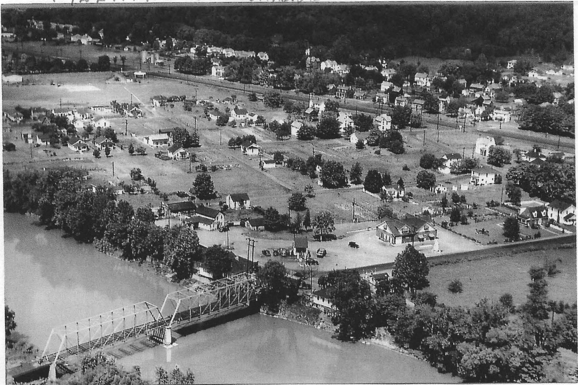
PILLING ST. BRIDGE
