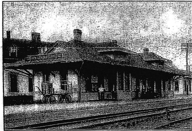
Photo courtesy of William Casteel With the railroad business expanding across the nation, Newcomerstown found the need for a larger, more efficient depot. Pictured here is the Union Station Depot that was constructed, and open to the public in August of 1899. The structure was later abandoned when the railroad fell out of popularity and was demolished by the Conrail railroad company in March 1981.
