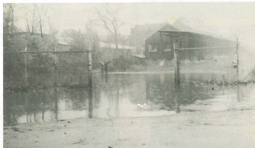
Flood waters cover the low-lands around the Eddy plant.
