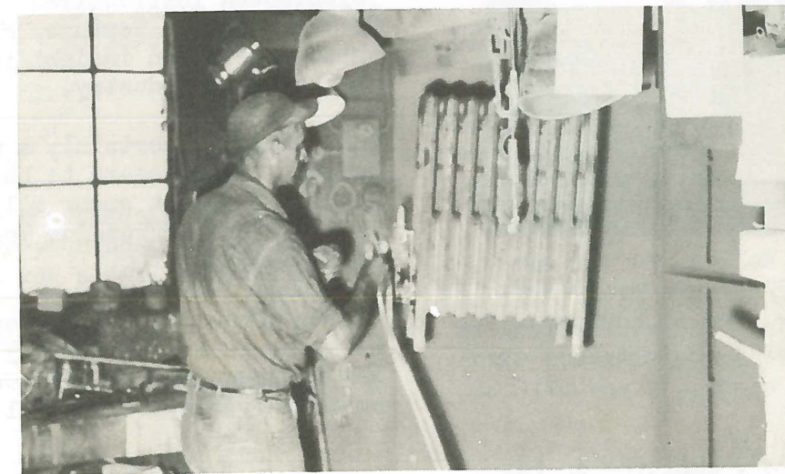
Above, center: Vernon Kail spray paints another radiator after it has left the assembly line.
