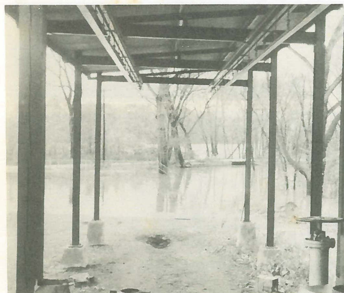
Another view showing flooded area near the plant.
