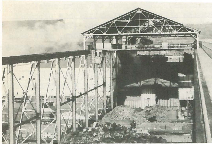
Here is a view of the charging crane runway, where scrap and pig iron are unloaded and stored.
