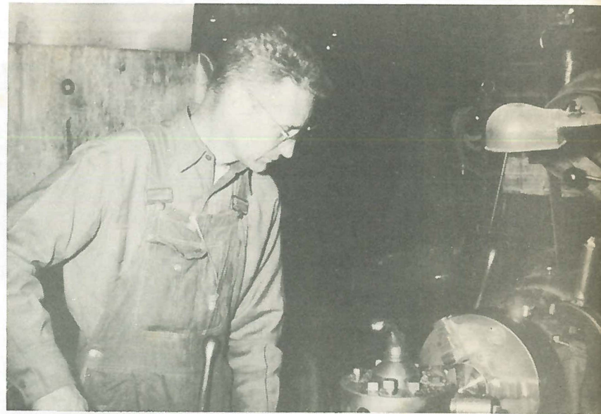
Wayne Lindly (above) operates the new abrasive cut-off machine. Wayne is tightening a new abrasive wheel preparatory to cutting brass rod. This machine is a marked improvement over our old method of cutting with a band saw.
