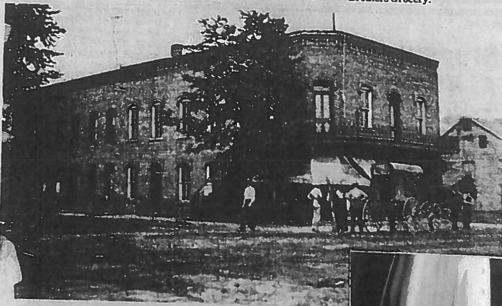
This was the site of Morgan's Pharmacy before it moved to its present location on College Street. The building had been a pharmacy since the turn of the century. A bowling alley was above the pharmacy.
