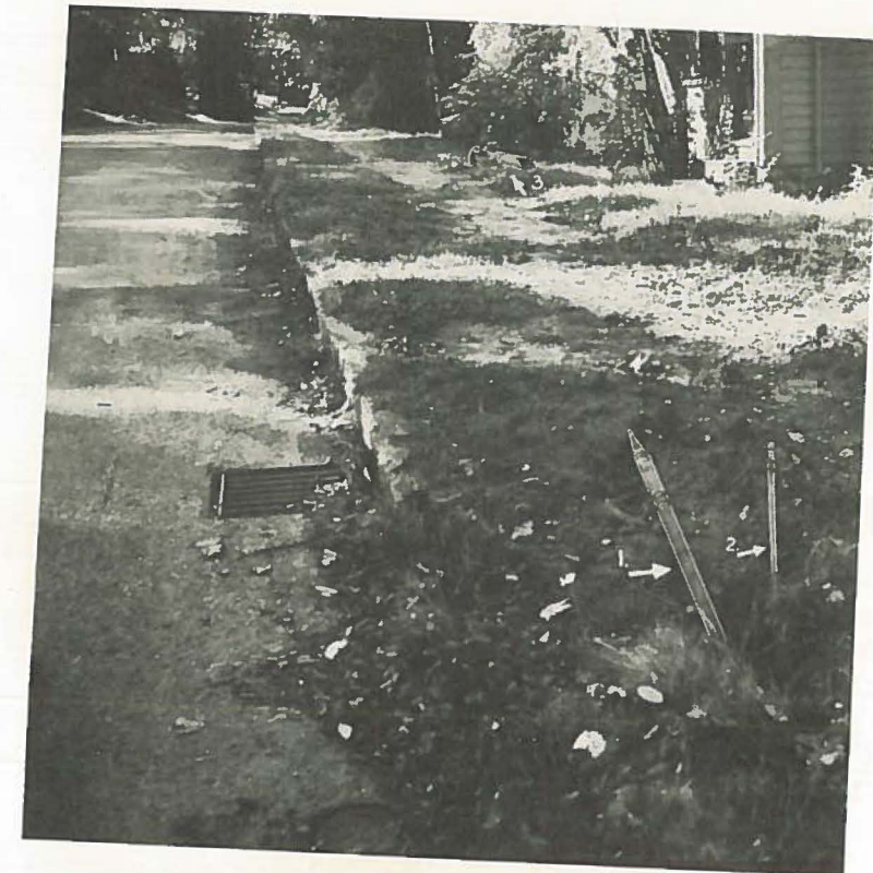
Damaged Eddy Hydrant
