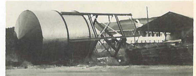
Here's the answer to the picture "What is it" that appeared in the last issue of the Clow News. Scotty Kelley took an inside view of the new tank.
