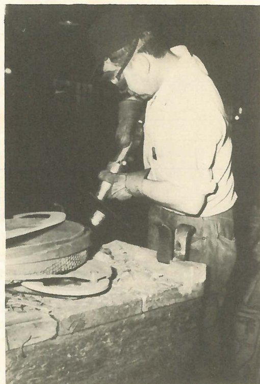
George Temple our Inspector was photographed doing a job grinding on a belltrap.
