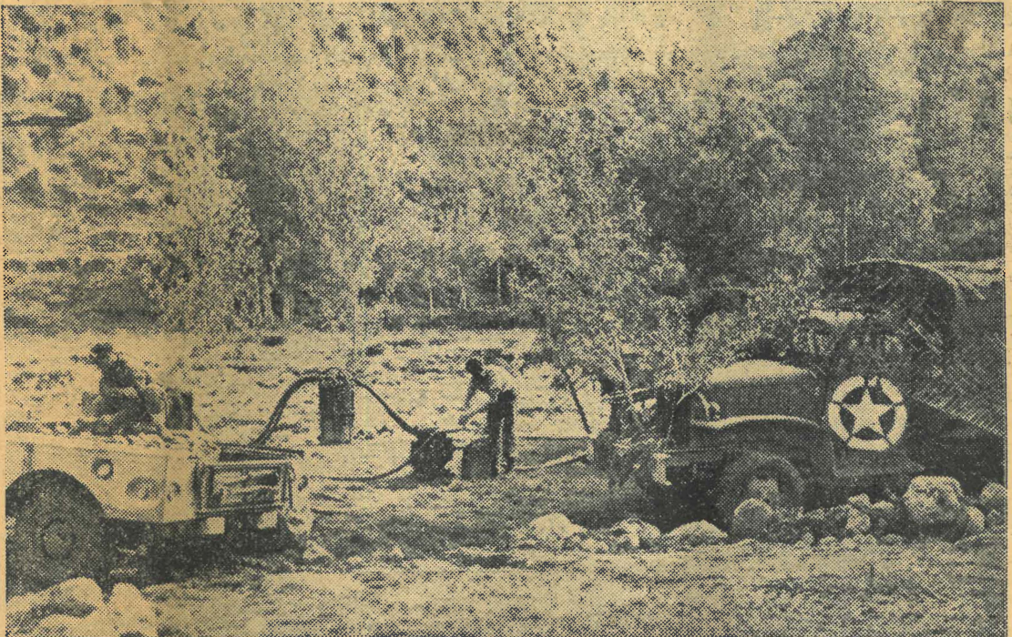
ENGINEERS PLACE THEIR EQUIPMENT beside a stream in Italy to keep purified water flowing constantly to units of the Allied 5th Army. Water from the stream is pumped through purifying filters and then into a canvas tank where it is held until needed. Water from any source, no matter how polluted, can be purified with equipment which moves with U.S. troops.
