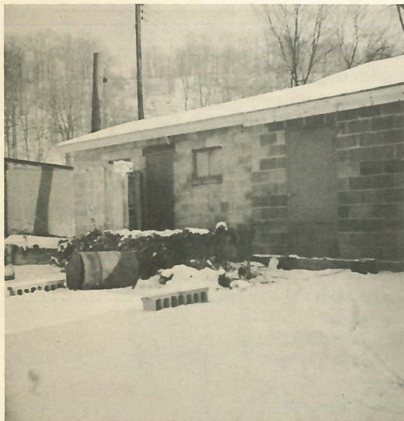
Clow Lodge building with debris left after flood (note water line on door).
