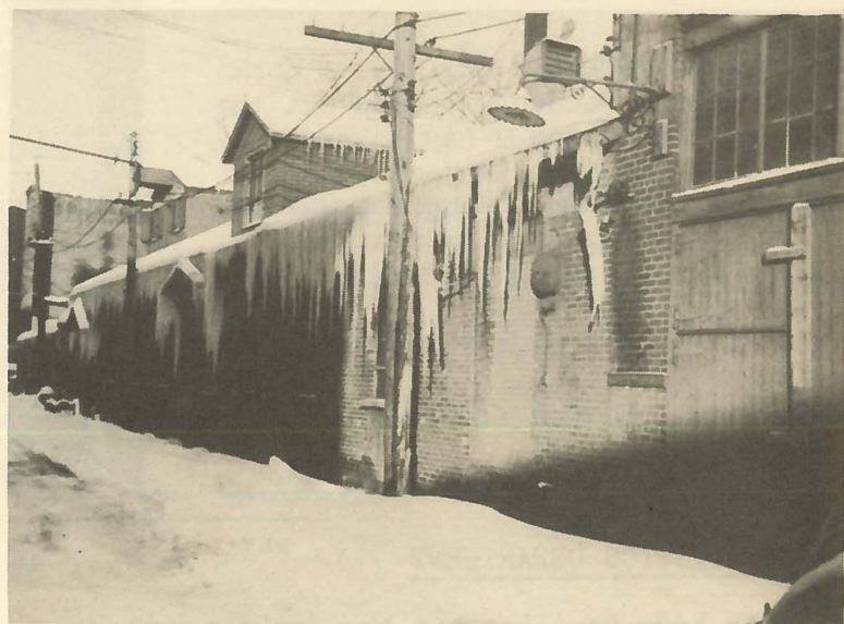
Along the Foundry Cleaning Department, looking toward the Brass Foundry.
