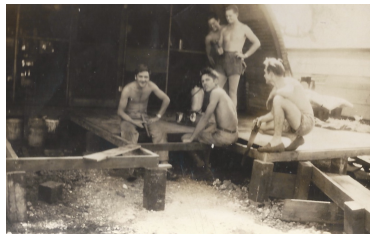
Building a Porch on Guam 1945
