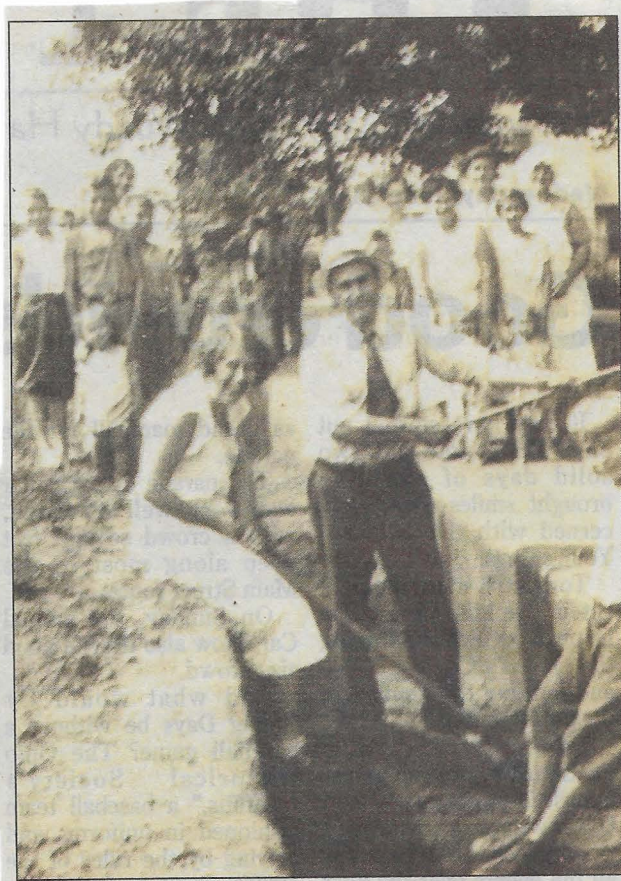
Newcomerstown residents, Ruth Cunningham, and John Jones are seen digging in a trench on south Mulvane Street following the discovery of several skeletons in August 1934. The photo was taken by the late Anna Sells who resided on Mulvane Street at that time.
