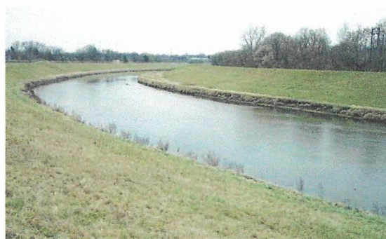
A channelized portion of the river in Massillon in 2006, as viewed from the towpath trail of the former Ohio and Erie Canal
