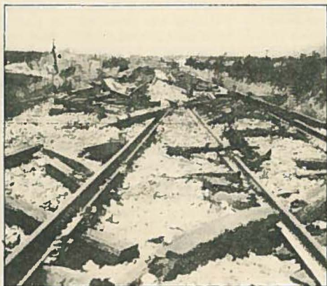
Destruction on the right of way.
