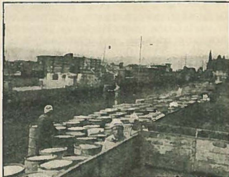
Arabs transferring load from standard gauge cars to the meter gauge cars at Ouled Ramoun.
