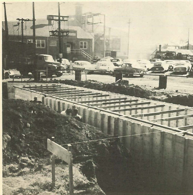
Forms we place for scale pit. Intruder proof, if you will recall the happening of a few years ago.
