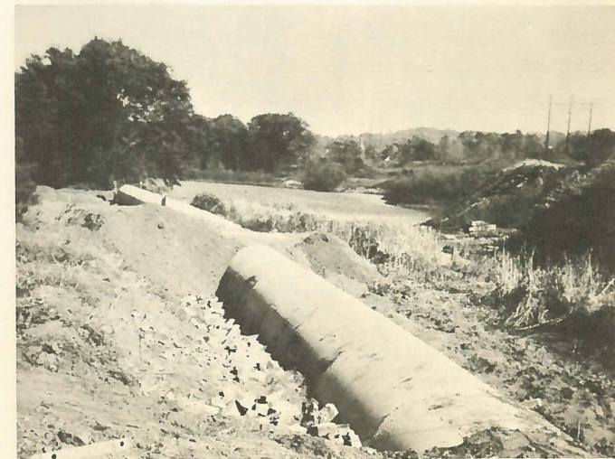
Extension of 48" drain lines at north end of plant.
