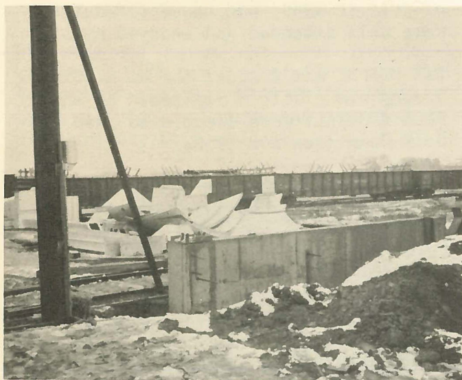
CONSTRUCTION PROGRESS ON CEMENT LINING BUILDING
