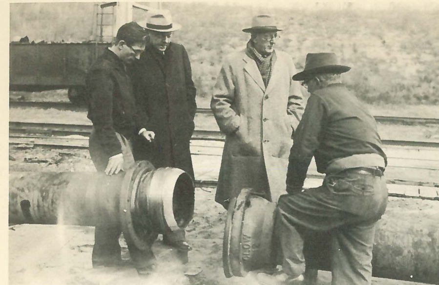
Jim Majors, George O'Day, W. E. Clow, Jr. and E. L. Bolen inspecting the new river crossing pipe. Still very much in the experimental stage, these pipe are designed for use in laying a line across a river.
