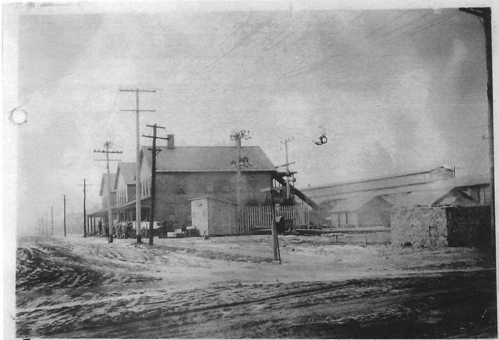
TEMPORARY CLOW SUBSTATION NEWCOMERSTOWN FEB. 23, 1924
