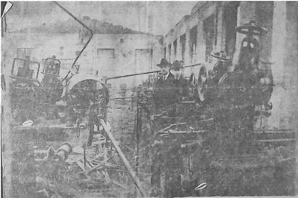
DISASTER STRIKES—Plant Supt. Frank Wilson and Russell Bean, son of a former perintendent, survey the damage at the Rex File Co. following the April 12, 1917.
