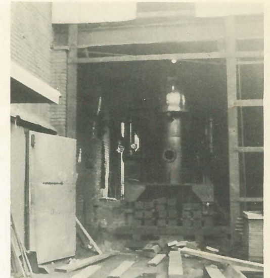
Melting section and windbox were moved through side.
