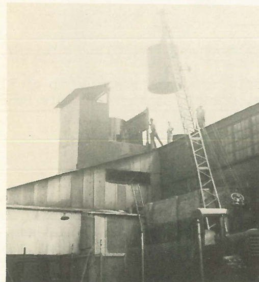
Last section being hoisted up.
