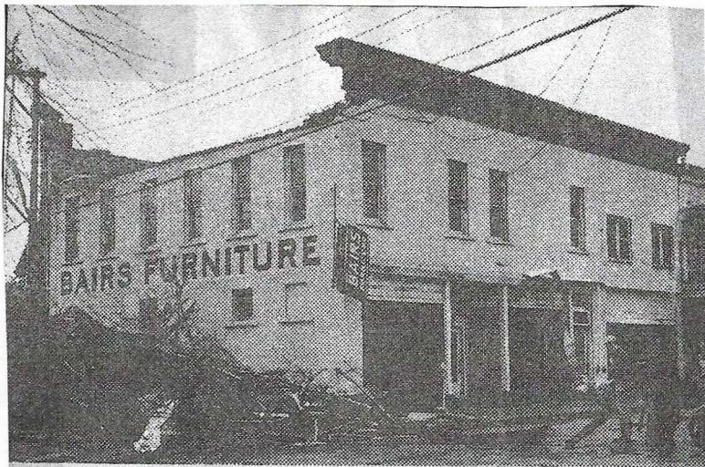
Tornado wreckage on Main St.
