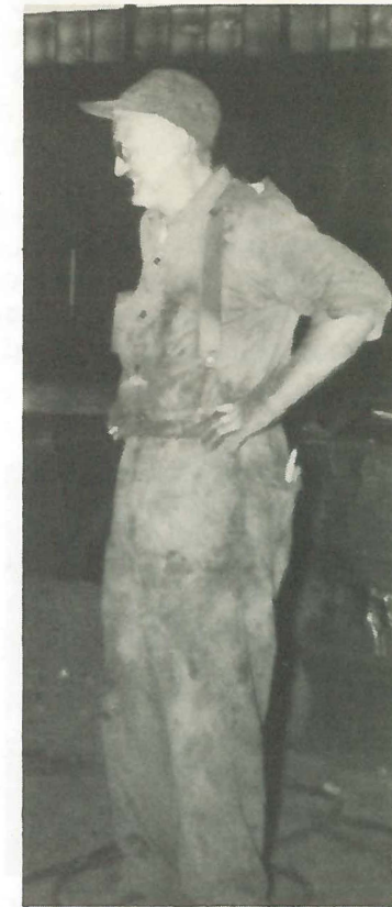
Red Young, of Maintenance took time out from an electrical wiring job to pose for this picture.
