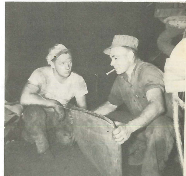
Richard Morrison and Arthur Courtright installing a new conveyor belt in the Molding Floor Department.
