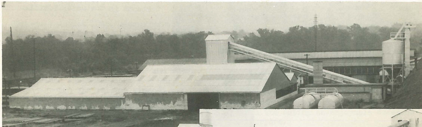
Above: General view of the new Cement Lining Plant at National.
