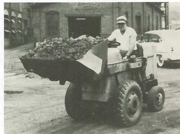
Leo Boone transferring a payload full of coke to the cupola.
