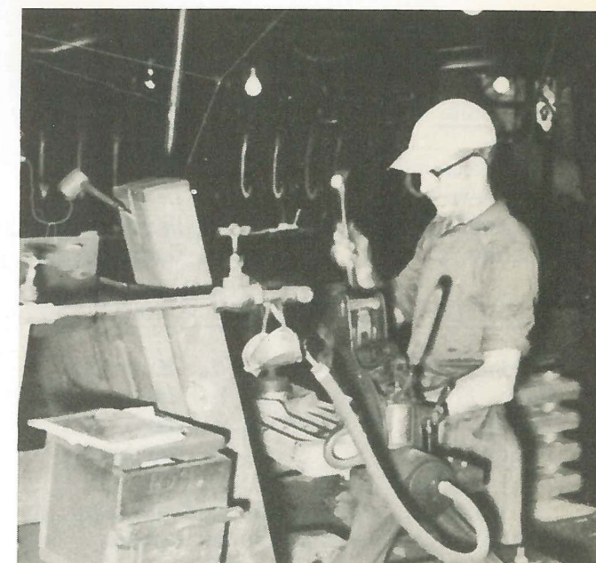
Bill Welsch, water testing a radiator loop. Bill was just recently recalled to work.
