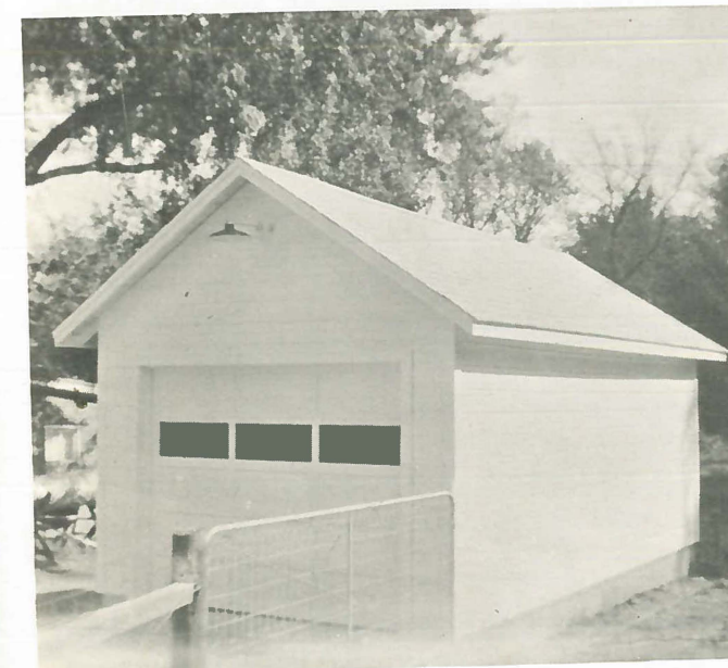
This miracle of miracles was submitted by LEROY WYMORE who bets that no one will recognize it as the last garage sold from Iowa Valve property. LEROY purchased the old building and during his summer vacation, helped to lengthen and rebuild it.
