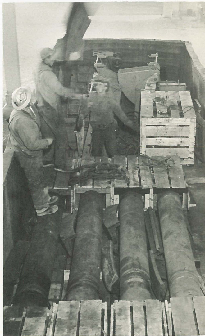
Being unloaded in this picture are casting machine cylinders (foreground); machine ladle stands; both interspersed with cupola liner plates, and other material fashioned by the Coshocton Plant.
