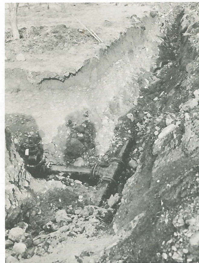
Photos above show pipe, valves and fittings being installed in glacial gravel, which underlays 2\frac{1}{2} feet of rich, black farm soil, which exists throughout this area.
