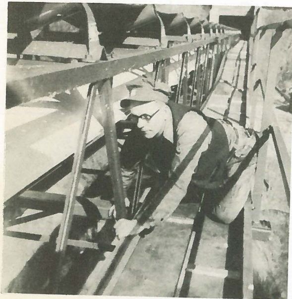
Electrician Gerald Bordenkircher checking on the first run of the new Core Floor conveyor.
