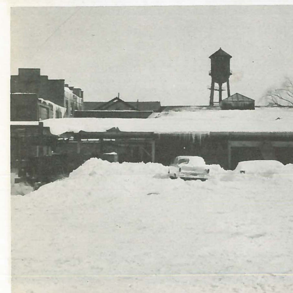
View of south parking lot.
