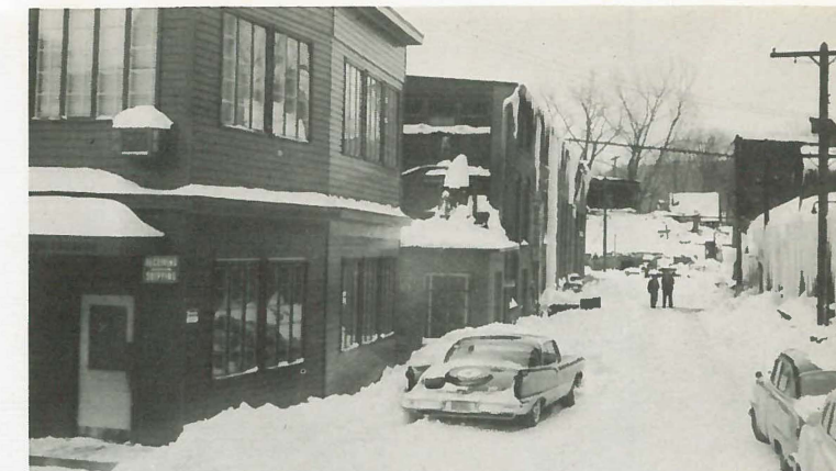
Main company street, showing offices and machine shop on left. Note hugh icicle on machine shop that extends thirty feet from roof to ground.
