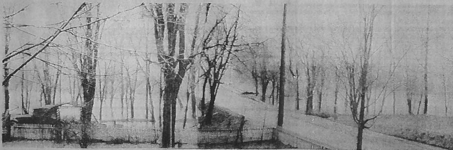
Bridge on East State Street
