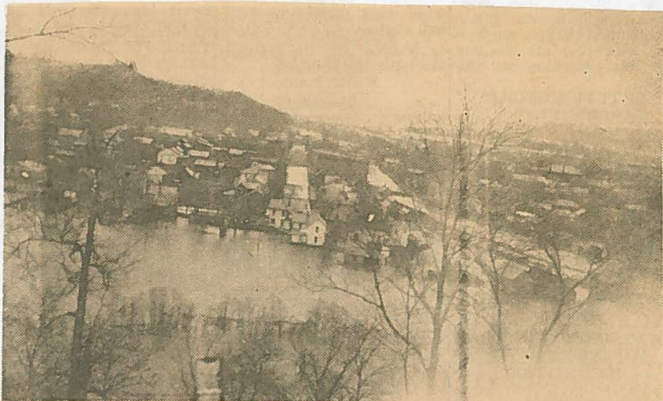
On Park Hill the view looked like this.
