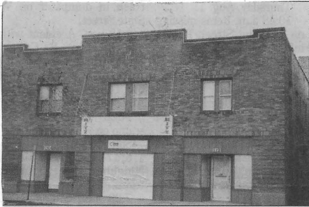
The Ritz Theater building as it appears today. The marquee, still intact, though vacant of the latest movie releases.
