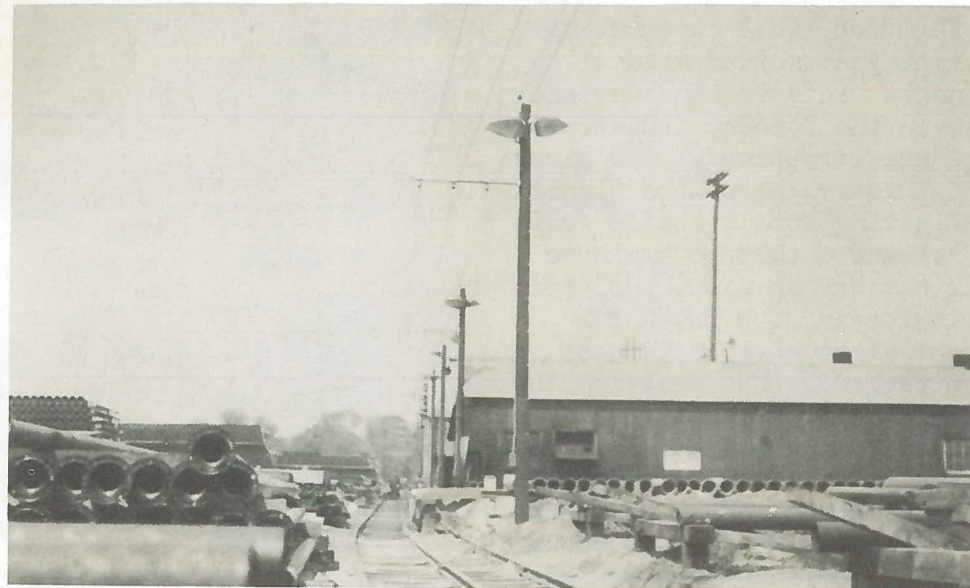
New lighting fixtures have been installed in the deLavaud Pipe Yards. This will eliminate many hazards that have been present in this work area because of poor lighting.
