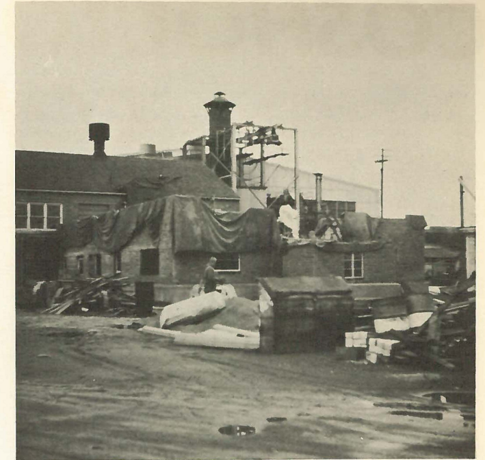
Progress on Laboratory extension.
