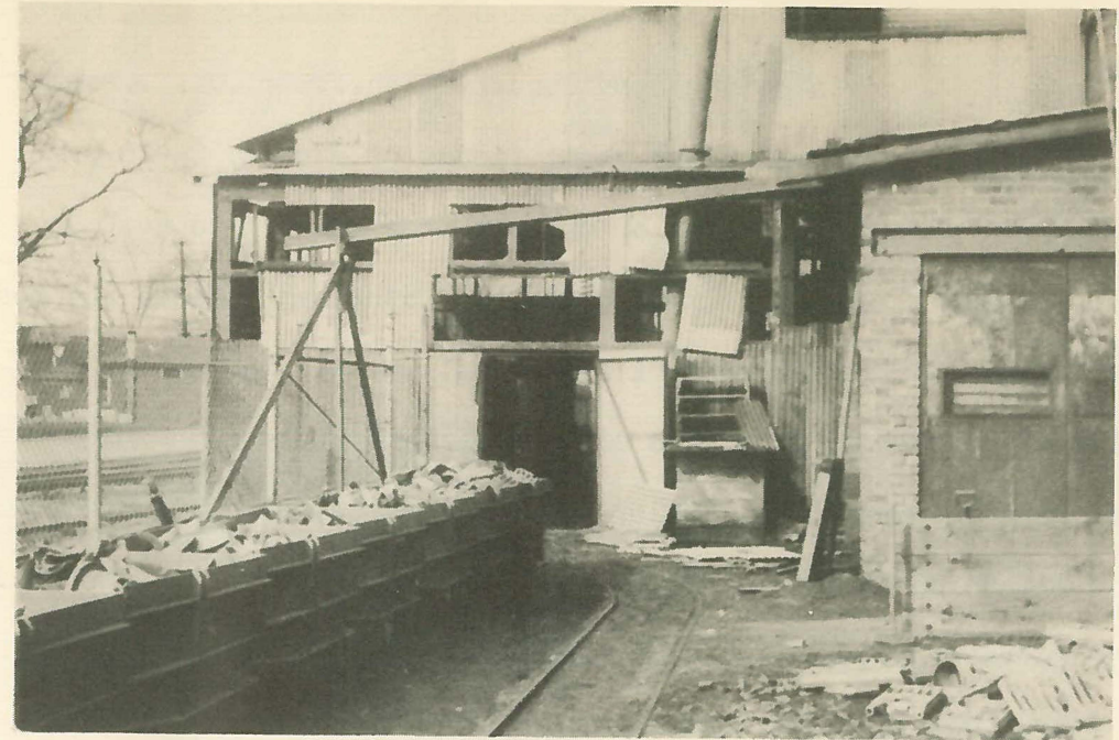
Looking at the south side of the cupola building. The doors were open at the time of the blast but all the other openings were blown there.
