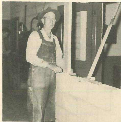
H. P. Clark working on an addition to the laboratory.
