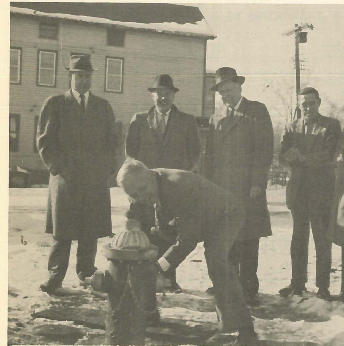
This group from Long Island is about to witness the smashing of a break-flange hydrant that has been installed in the earth to the pavement line. In the background, out of view, is a truck waiting for the signal to smash into this hydrant.
