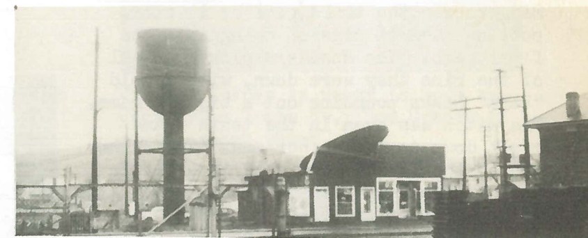
The top of the Pennsylvania Railroad's water tower was blown off and landed on this grocery store across from the plant.
