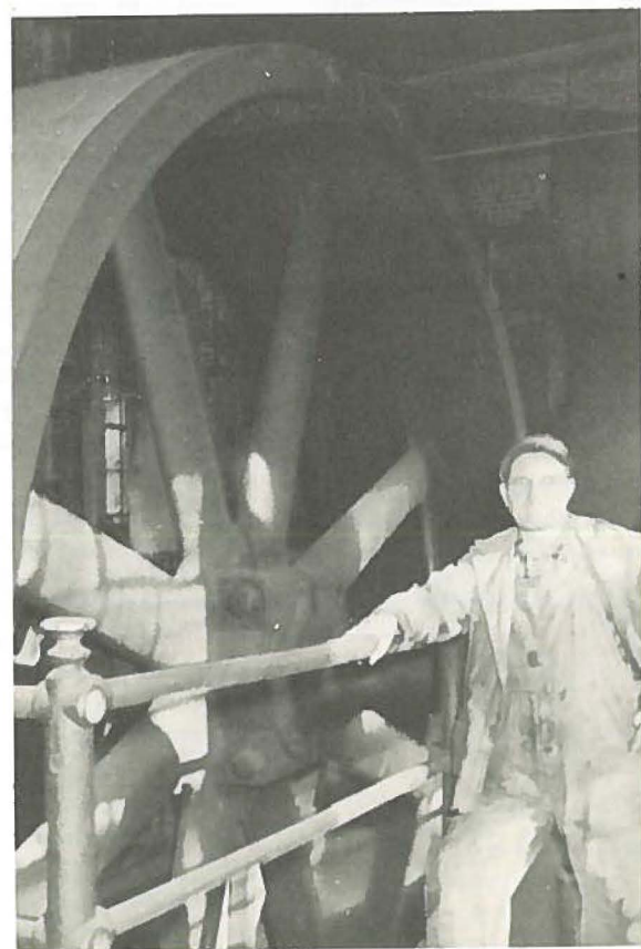
Hank Moss, fireman at Eddy, stands next to the big wheel of the air compressor in the Boiler Room at the plant.
