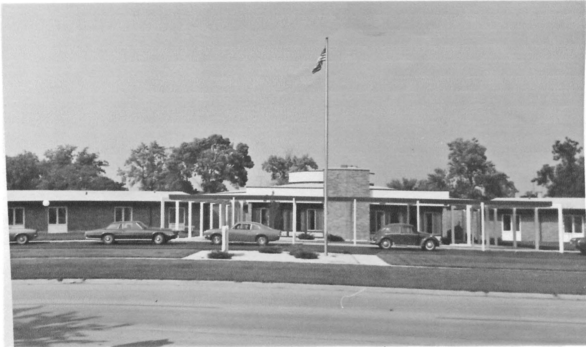
WEST ELEMENTARY SCHOOL 517 S. BEAVER ST.
