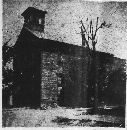
SECOND LUTHERAN BUILDING —This frame church was built in 1869-70 at a cost of $3,500 by the Lutheran parishioners.
