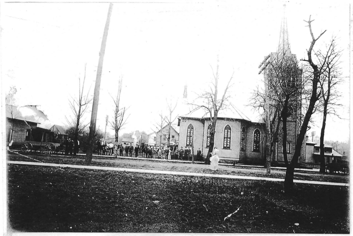
M.E. METHODIST CHURCH S.W. CORNER OF CHURCH & RIVER ST
